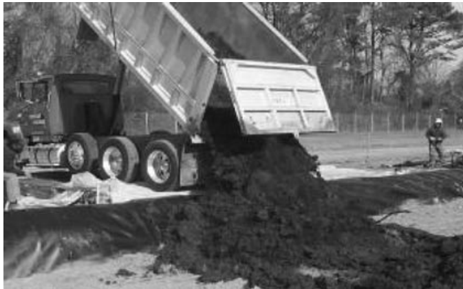
Exhibit 1. Placement of soil into treatment cell
