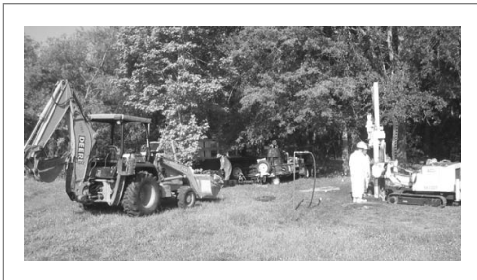
Exhibit 9. Application of EHC slurry using direct injection
