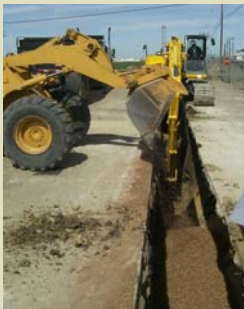
Figure 1. Placement of EHC and sand mixture into excavation trench.
